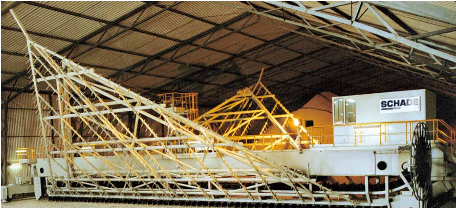
Bridge-type Reclaimer for homogenization
