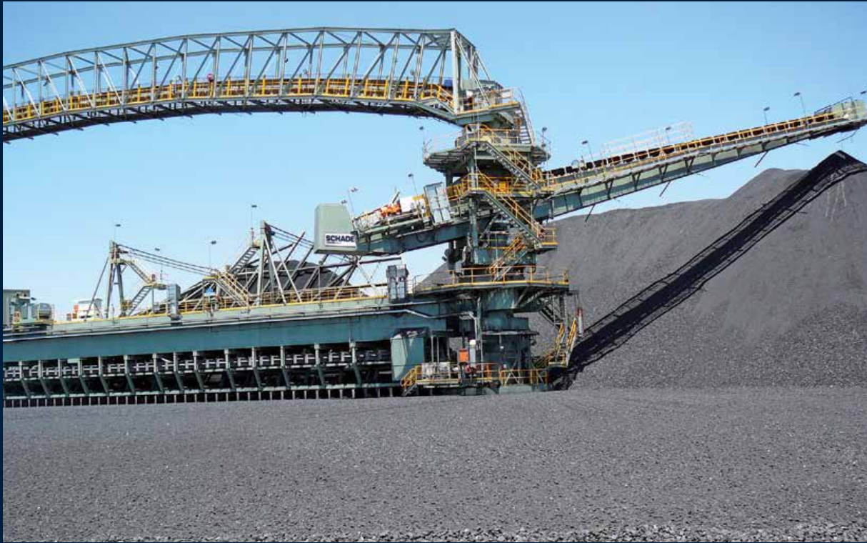
Circular Blending Bed for outdoor operation
