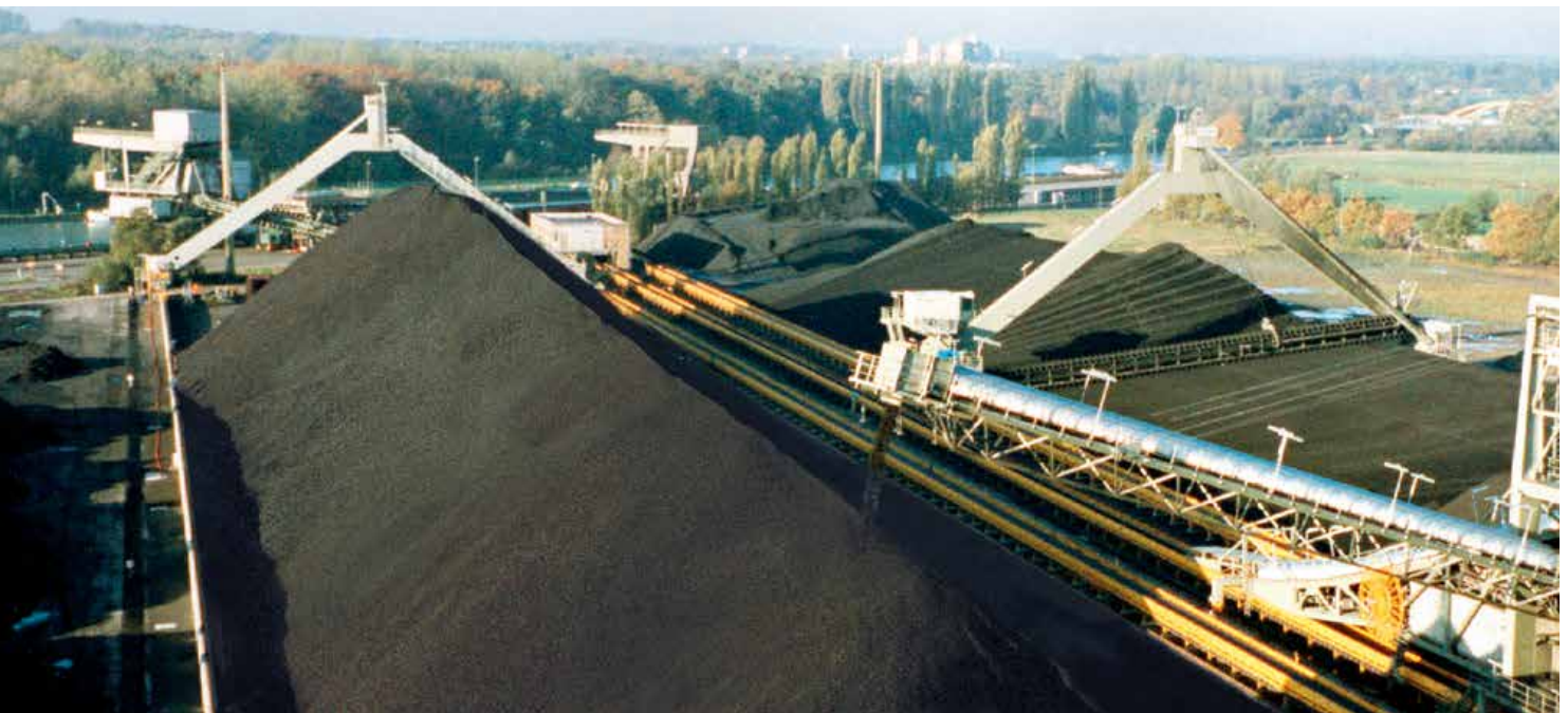
Portal Scraper Reclaimers with Stacker
